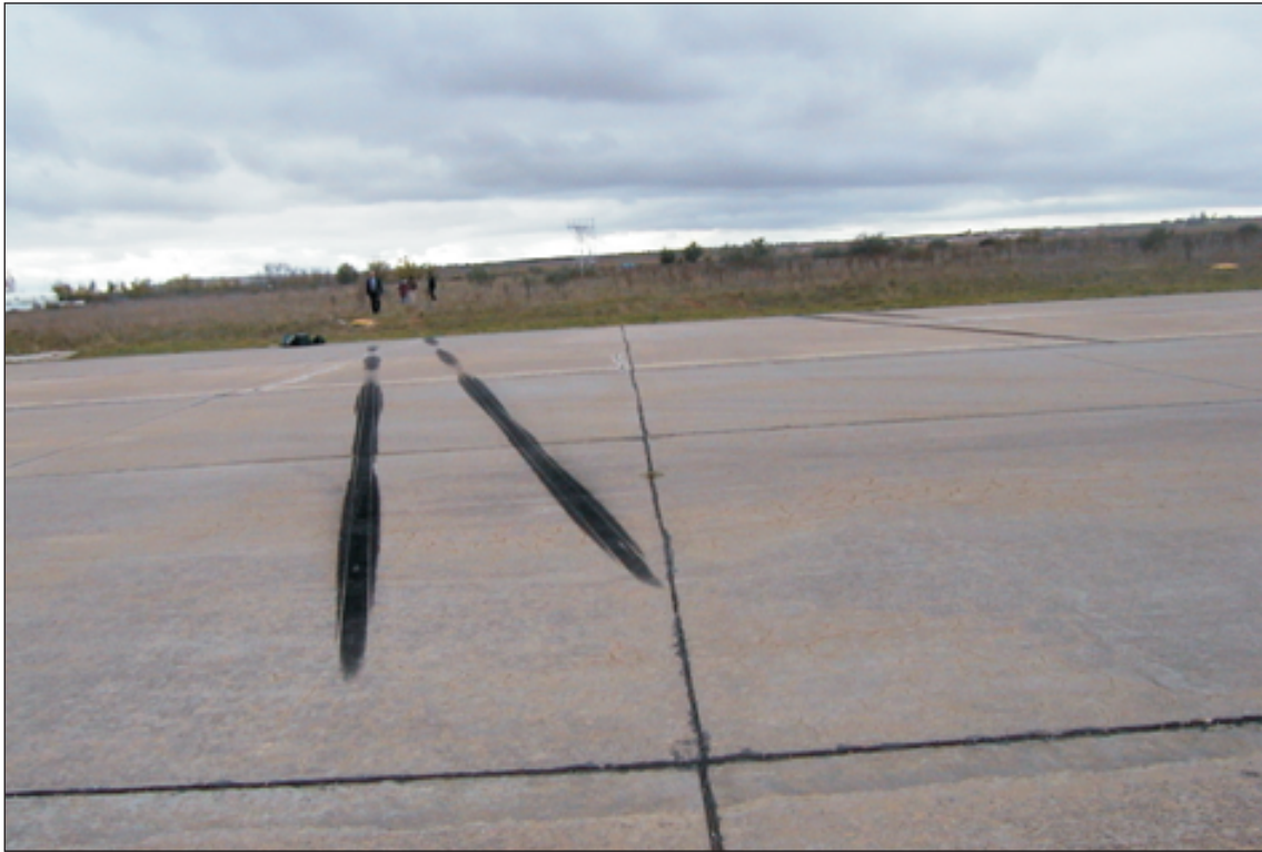
General view of the tracks over the apron
