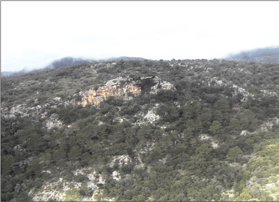
Figure A-1. Panoramic view of the accident site
