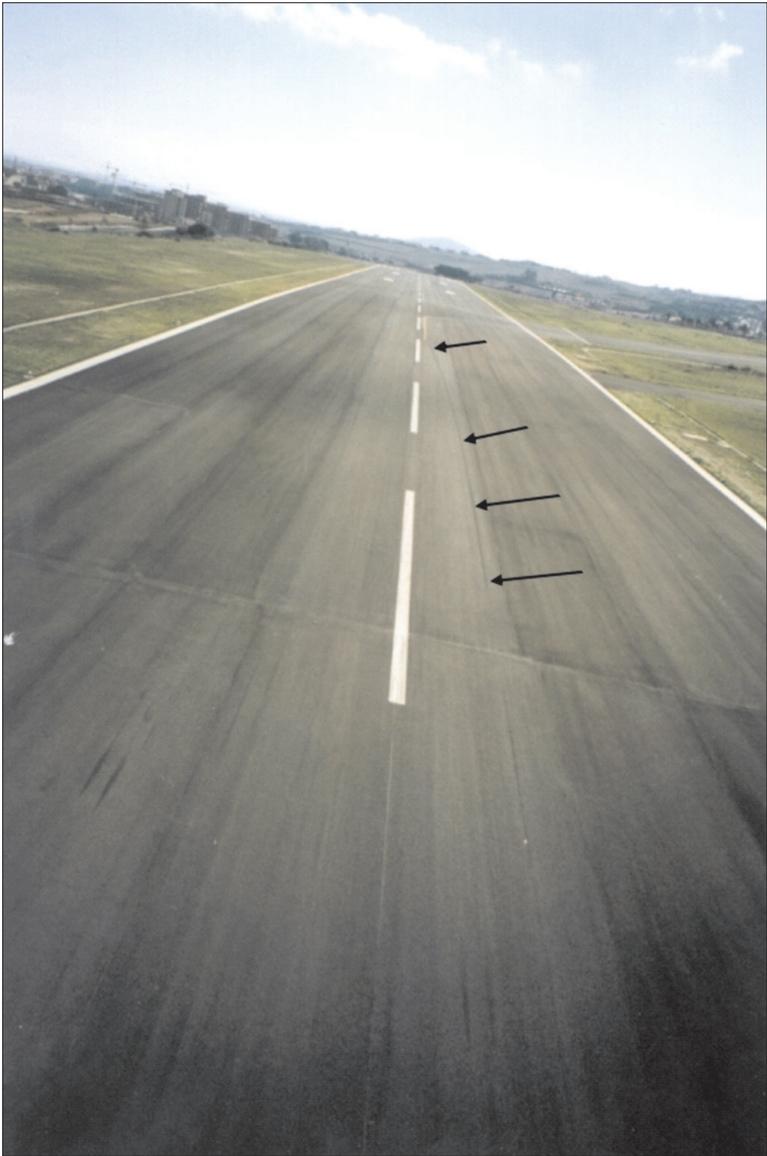
Photo 2. View in the sense of the landing roll. Track of wheel 3 crosses the runway axis
