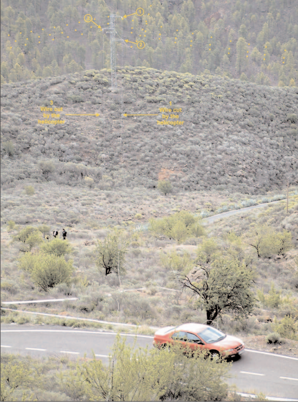
Figure 1.16.4. Lower tower. Wire 2, highlighted with yellow dots, remained undamaged. Lateral wires are also highlighted with yellow dots.
