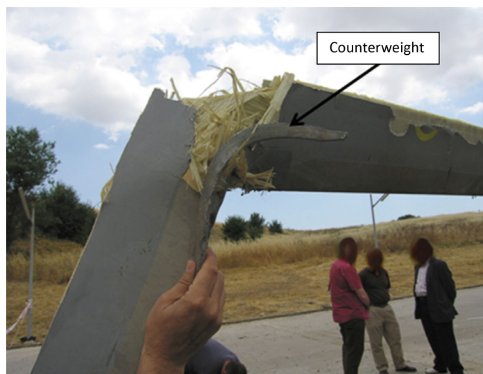
Figure 5. Red blade. Close-up of detached counterweight
