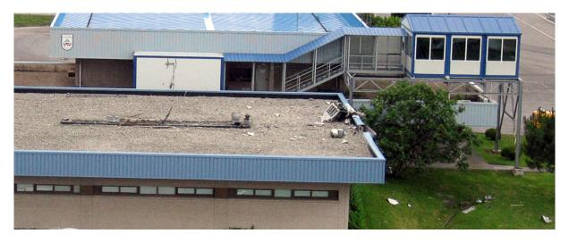
Figure 2. Photograph of damage to the services building roof
