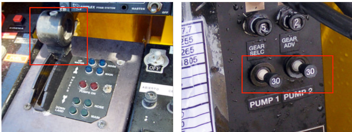
Figure 2. Gear lever in the UP position and tripped gear pump breakers
