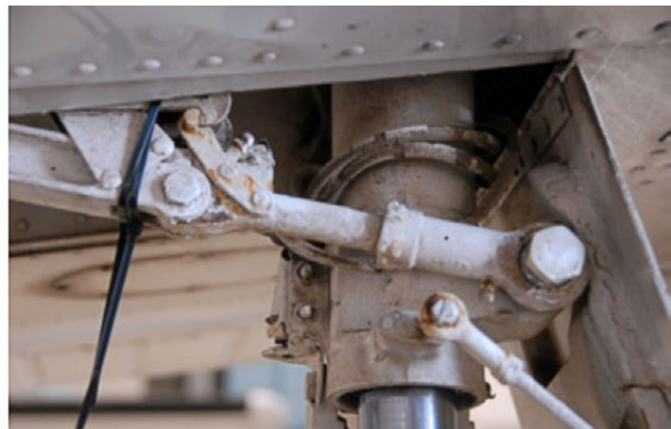
Condition of the left gear leg locked in place with a flange
