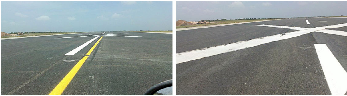
Figure 2. Landing marks, first from right gear and then from left, near the fourth runway-closed marking
