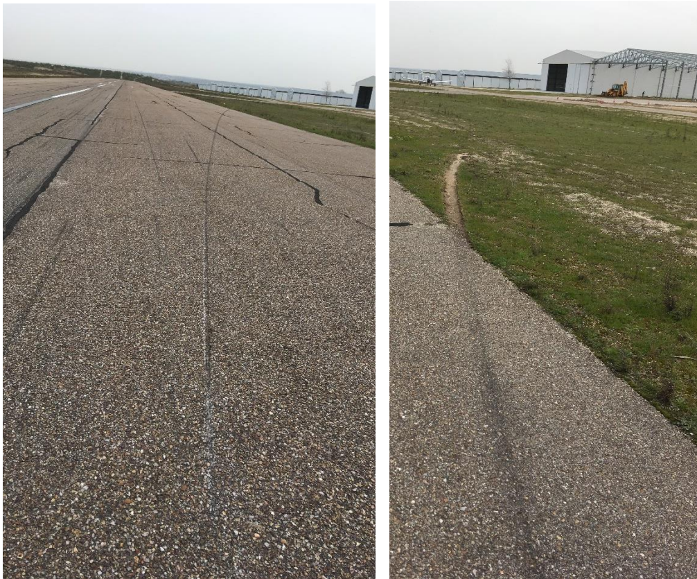
Figures 5 (left): mark on the asphalt; and 6 (right): mark on the edge of the runway and the mud and grass side strip
