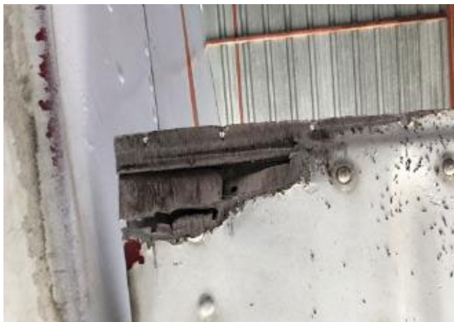
Photograph 8. Underside of the right flap
