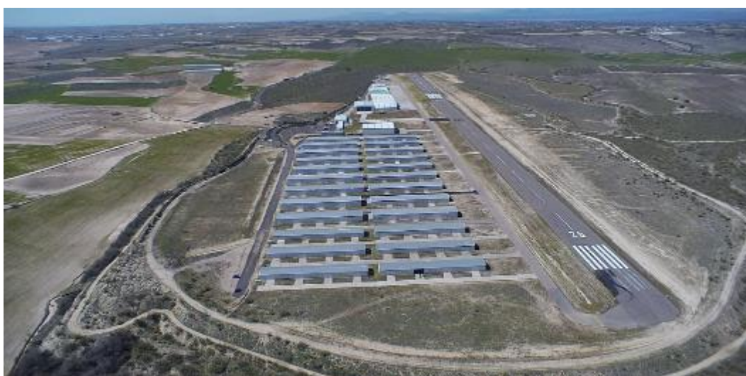
Photograph 5. Casarrubios del Monte Aerodrome
