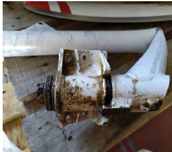
Photograph 16. Lower part of the nose gear leg that dragged along the runway
