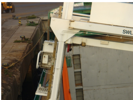
Photo 6: Bent hooks on the port side.
