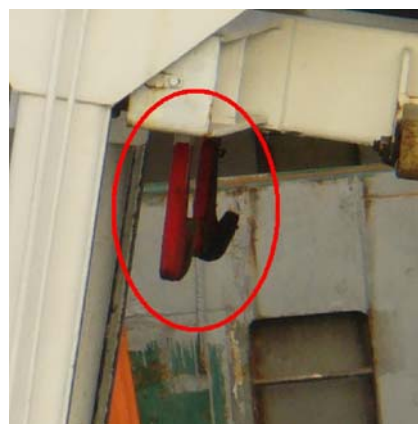
Photo 7: Enlargement of bent hooks.
