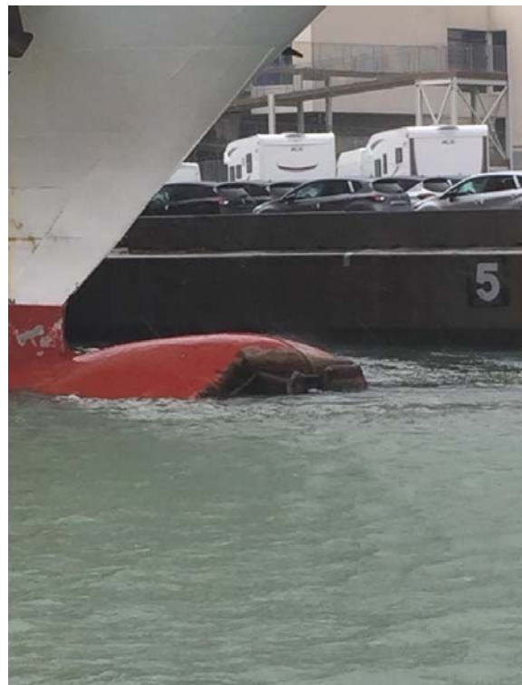
Figura 10. Damage to the bulbous bow
