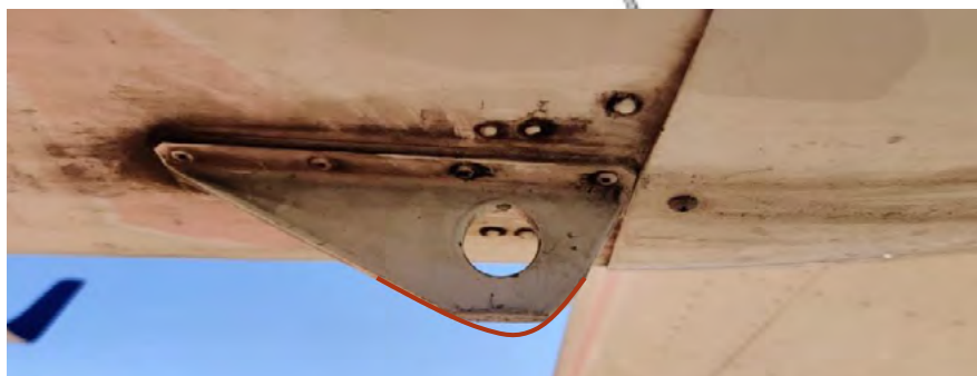
Photograph 19. Tie-down ring on the underside of the tail cone
