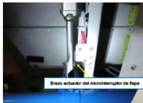
Photograph 27: Flap position microswitch of the gear warning system
