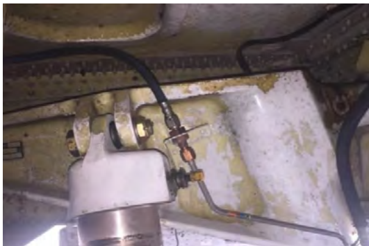
Photograph 10: hydraulic fluid lines
