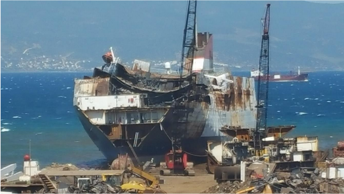
Pic 1: M/V SORRENTO – Initial phases of demolition (21 apr 2016)
