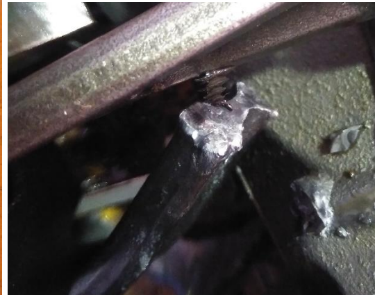
Figure 11: Close-up of connecting rod rupture (body end).
