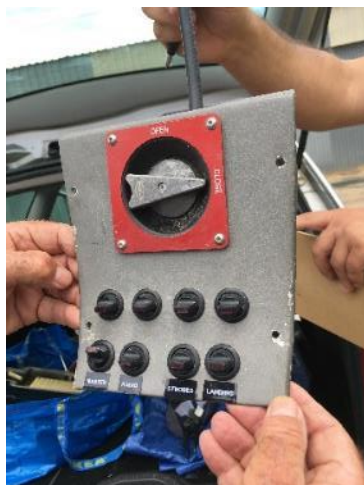
Photograph 15. Fuel shut-off valve
