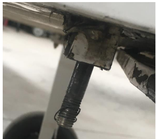
Photograph 9. Material wear to left leaf spring to fuselage lateral attachment bolt
