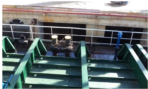
Figure 3.3– Port Side Overflow
