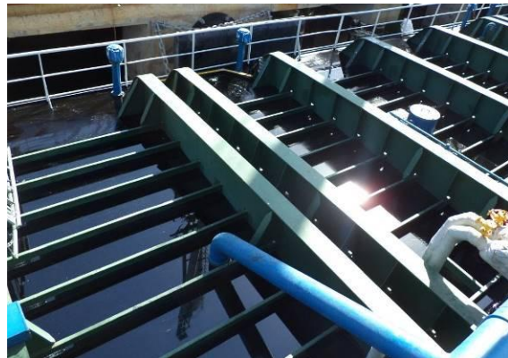
Figure 3.5– Port Side Overflow
