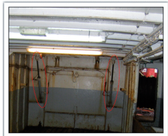
Figure 25. Fastening hardware for the door used for accessing the fish processing area from the upper deck
