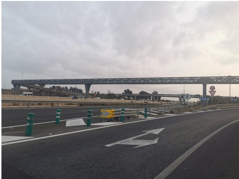
V-21 p.k. 14+500 pasarela peatonal
