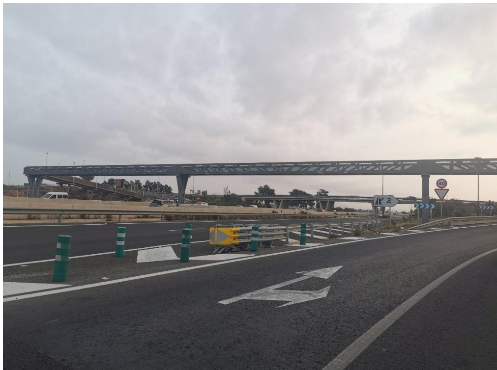
V-21 p.k. 14+500 pasarela peatonal
